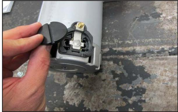
4. Pull the brush and spring assembly out.
