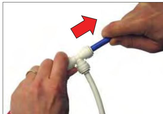
5. Test the fitting / hose connections for leaks prior to leaving the site.
