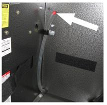
5. Place a suitable container under the end of the oil drain hose.
