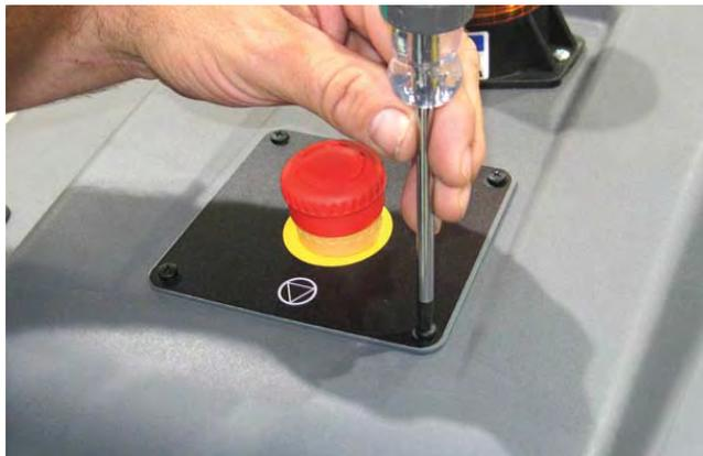
4. Carefully pull the E-Stop button assembly from the recovery tank cover. Do Not break or damage wire/cable connections when pulling the E-Stop button assembly from the recovery tank cover.
